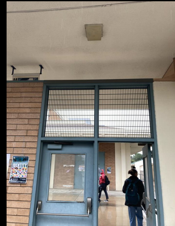
3. Grating above doors that access the Art courtyard in the middle of bldgs. 24, 25, 26, 27
