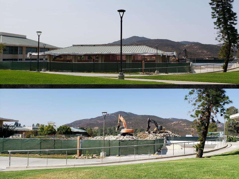
The concrete will be crushed down to <sup>3</sup>/<sub>4</sub>" in size. It will then be recycled and placed around the athletic fields
